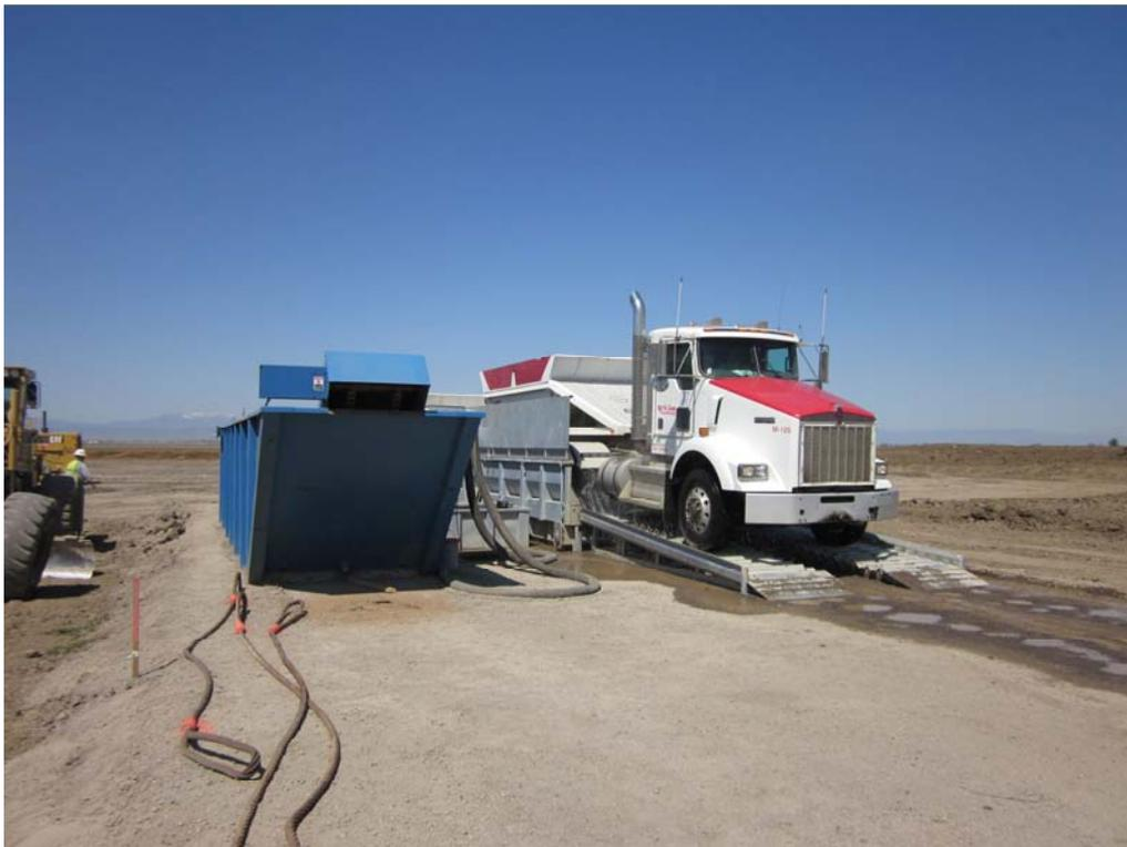
**Photo 6:** A tire washer and rattle plate are being utilized onsite for trucks exiting the remote well pad site and entering McAusland Road in order to minimize track-out.
