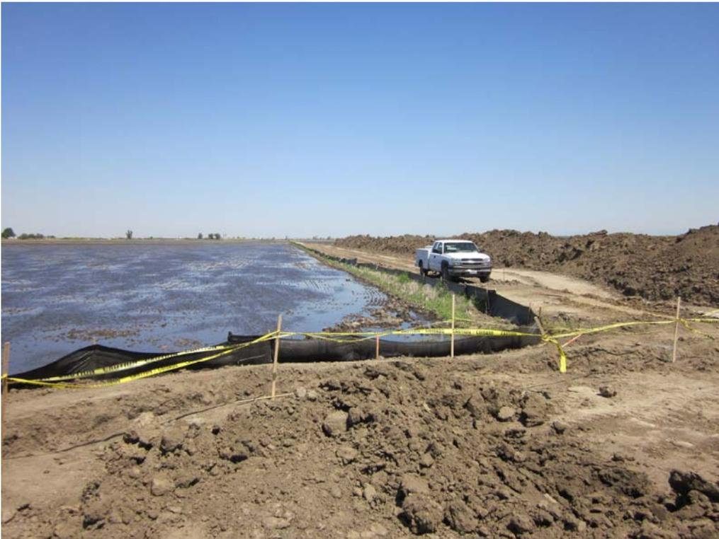
**Photo 4:** Silt fencing is placed along the perimeter of grading activities at the compressor station to minimize the potential for sediment to be discharged beyond the work limits.
