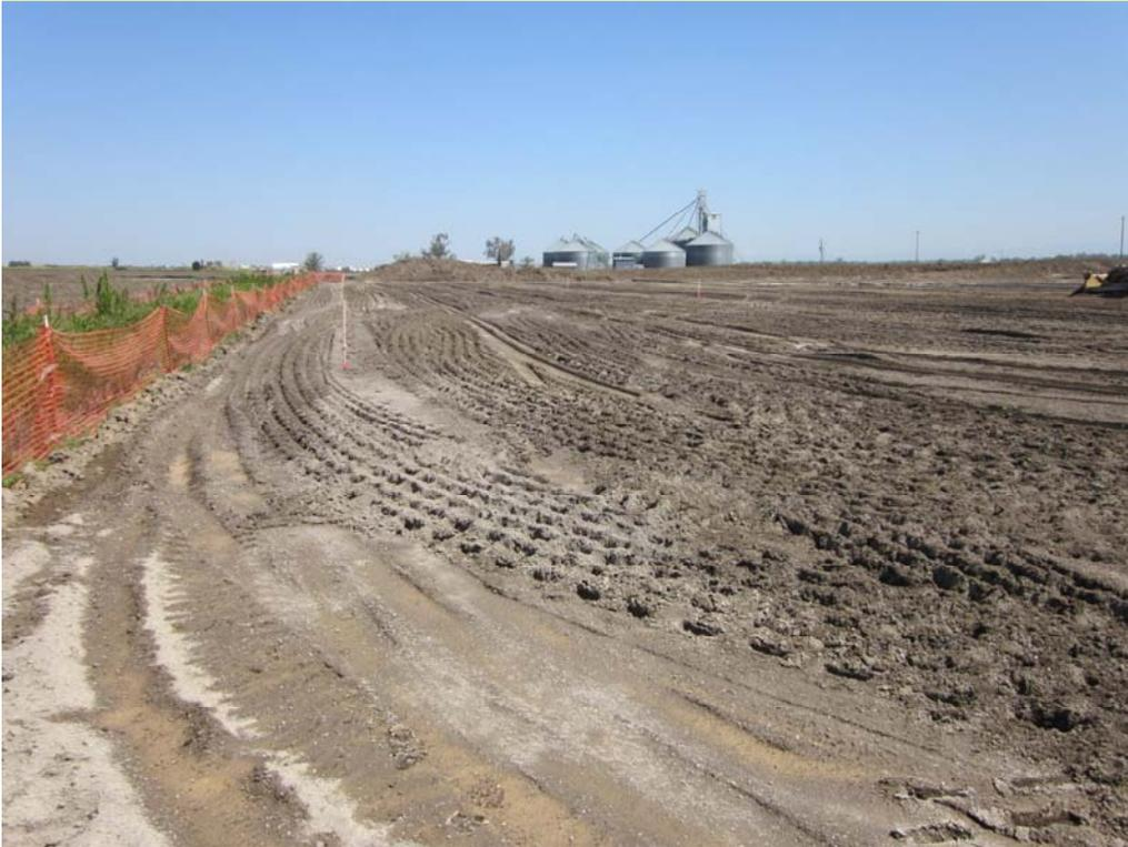
**Photo 1:** Construction crews complete soil compaction at the remote well pad site to obtain final grade.
